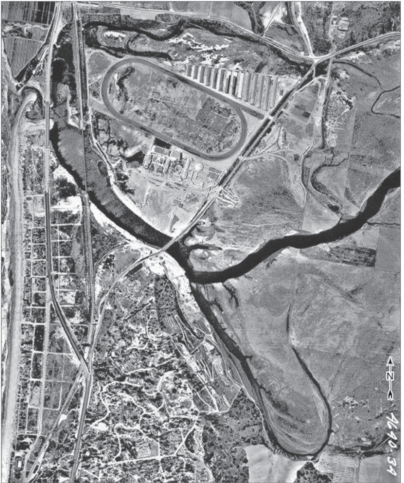
Figure 1-6. Aerial View of the Western End of the Project Area Taken in 1937
