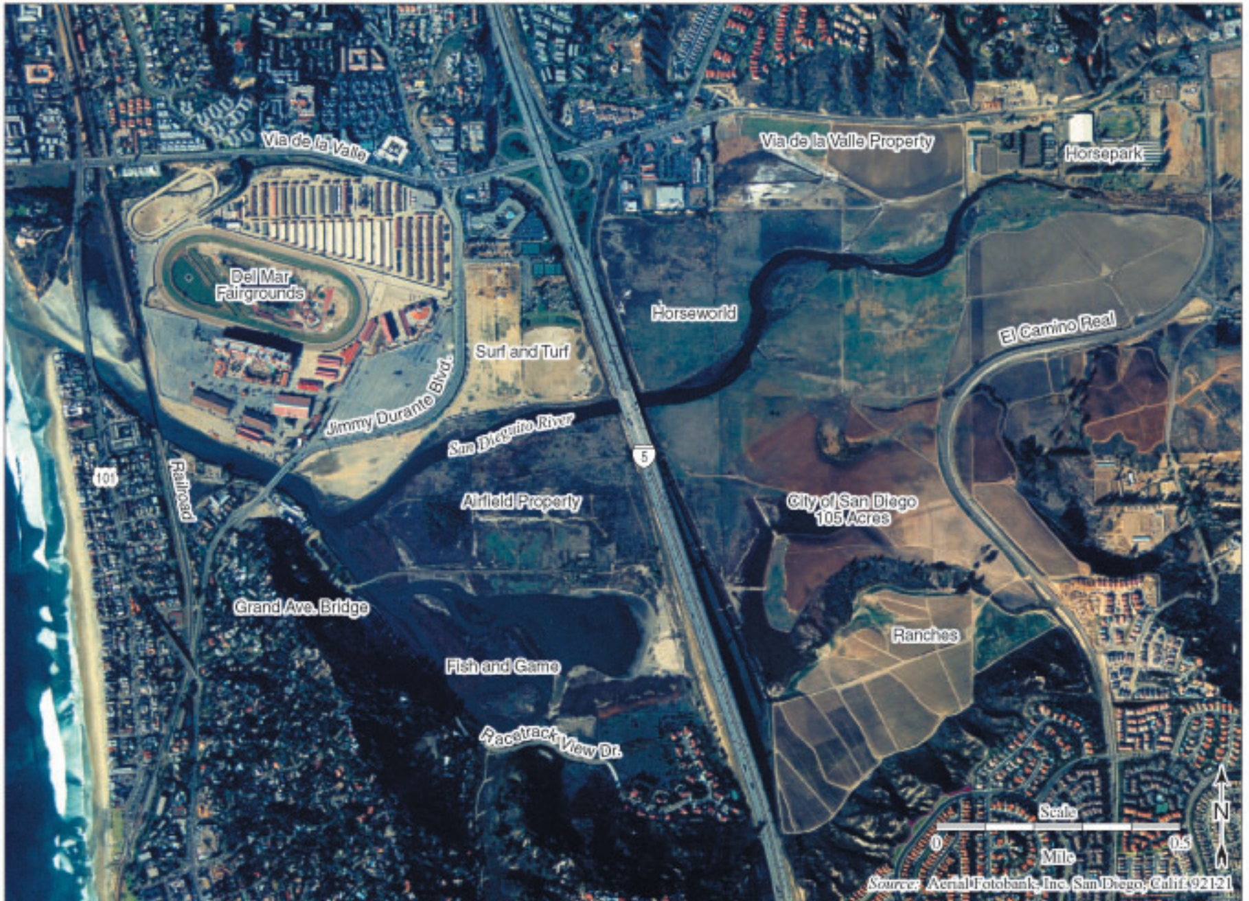
Figure 1-3. Aerial View of the Project Area
