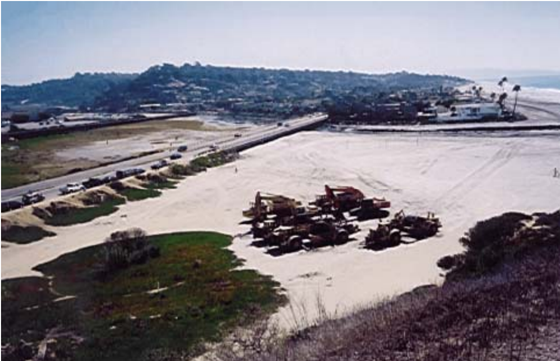
Figure 8-2. Staging area west of Highway 101 Bridge.
