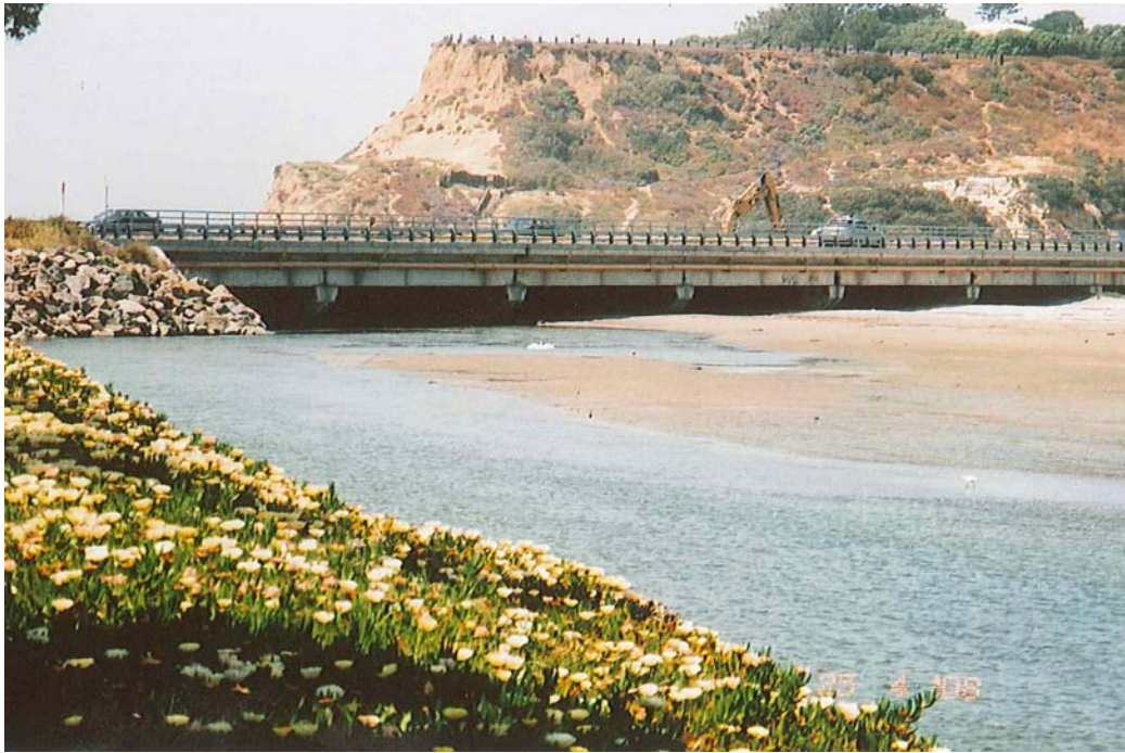
Figure 2-4. Photograph of Highway 101 Bridge looking west.
