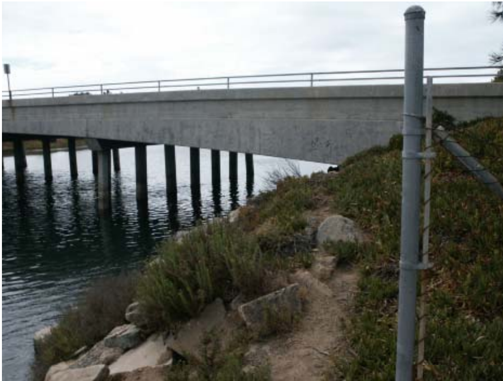
Figure 2-6. Photograph of Jimmy Durante Bridge looking east.
