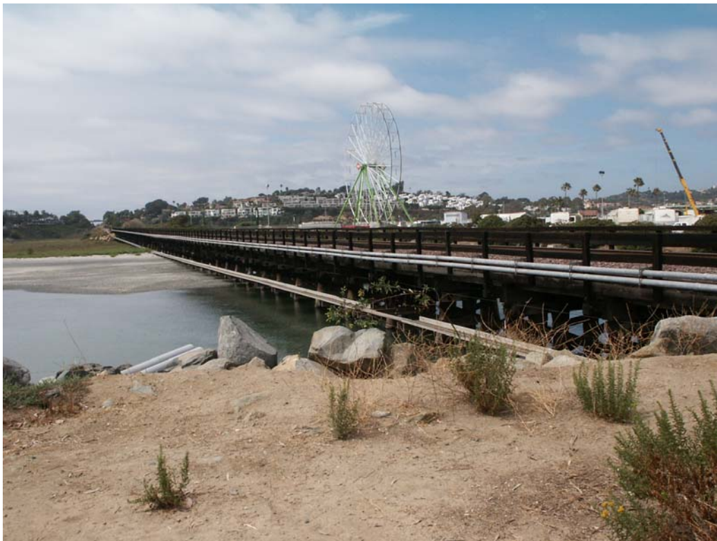
Figure 2-5. Photograph of Railroad Bridge looking east.
