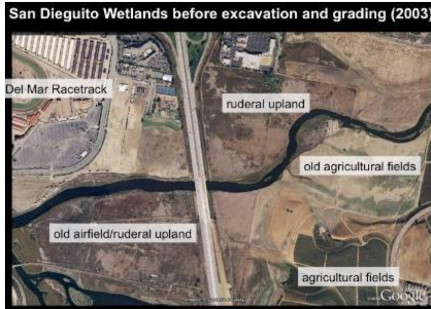
Figure 3.0.4a. Satellite view of the project site in 2003 before excavation and grading, including ruderal upland areas, an old WWII dirigible airfield, old agricultural fields, and visible at the bottom of the image, a portion of the Fish and Game Basin constructed in 1978. Image Source: Google Earth; U.S. Geological Survey.
