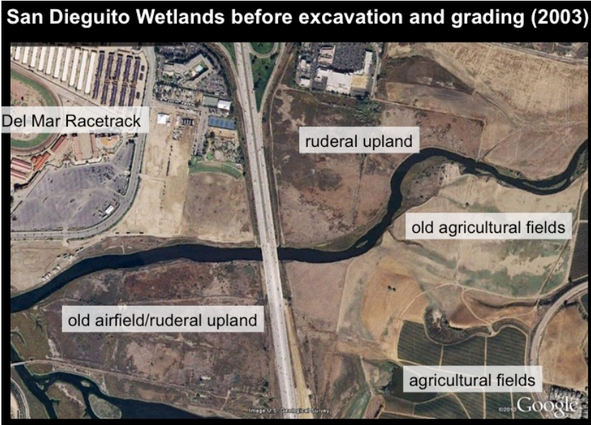
Figure 3.0.4a. Satellite view of the project site in 2003 before excavation and grading. Highlighted are the San Dieguito River and adjoining ruderal upland, including the site of an old WWII dirigible airfield, old agricultural fields, and visible at the bottom of the image, a portion of the Fish and Game Basin constructed in 1978. Image Source: Google Earth; U.S. Geological Survey.
