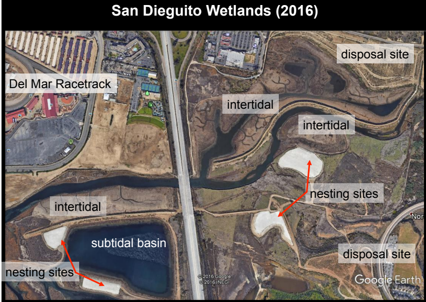
Figure 3.0.4b. During construction, the ruderal areas, old agricultural fields, and the WWII airfield were excavated and graded to create the planned intertidal and subtidal wetland habitats of the restoration project visible in this image taken in 2016. Image Source: Google Earth; NEGI.
