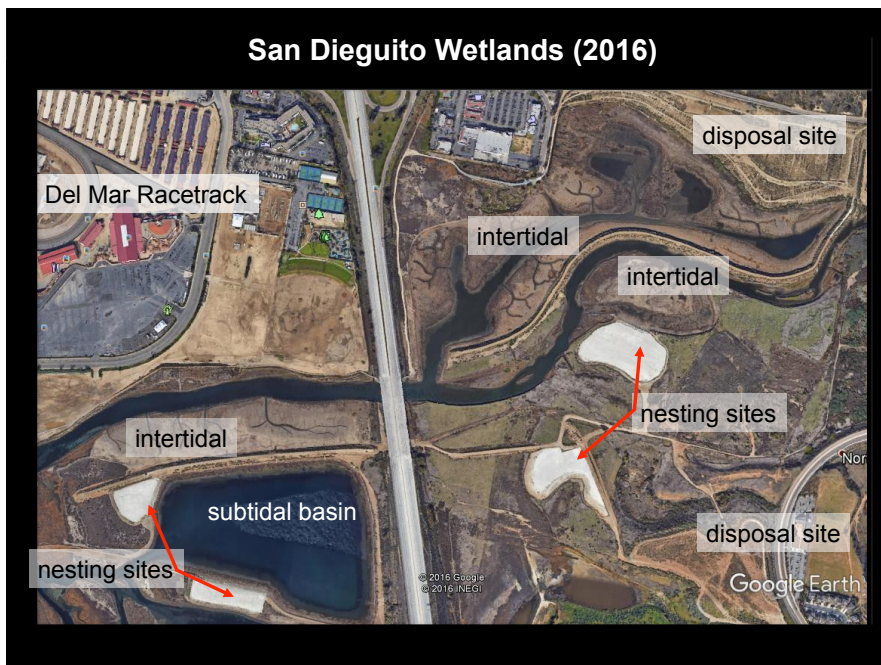
Figure 3.1.3b. During construction, the ruderal areas and old agricultural fields were excavated and graded to create the planned intertidal and subtidal wetland habitats of the restoration project visible in this image taken in 2016.
