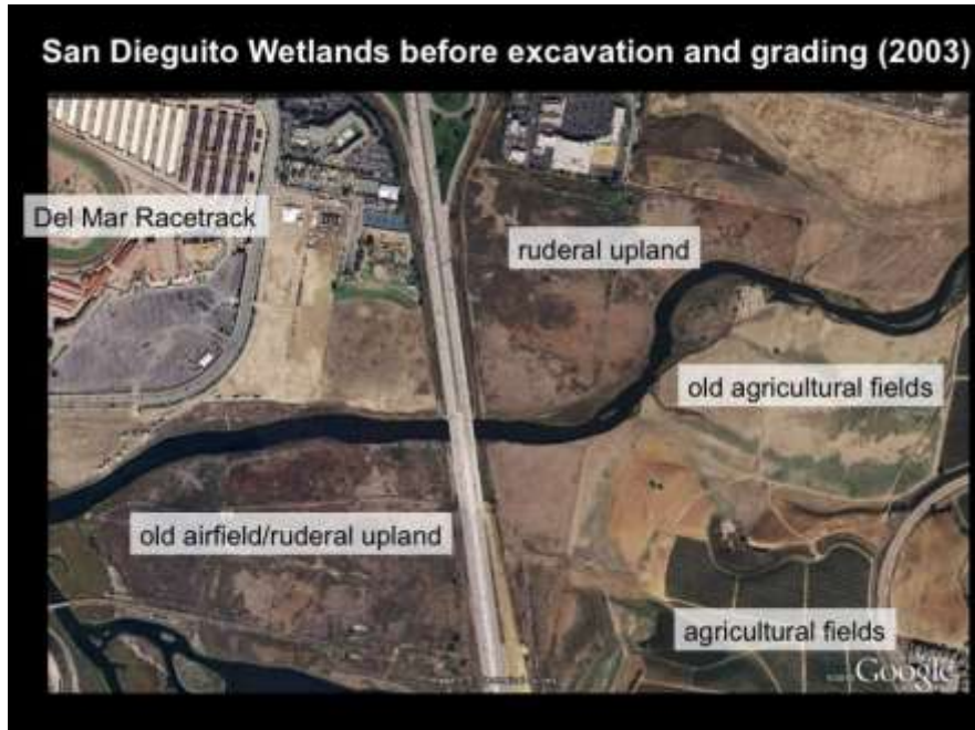
Figure 3.1.3a. Satellite view of the project site before excavation and grading. Highlighted is the San Dieguito River and adjoining ruderal upland, including the site of an old WWII dirigible airfield, old agricultural fields, and a portion of the Fish and Game Basin constructed in 1978 visible at the bottom of the image.
