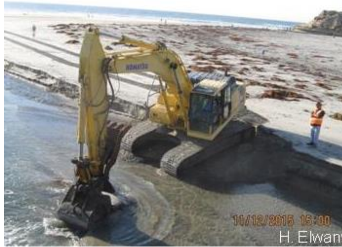
Figure 3.2.7. Dredging of the inlet at San Dieguito Wetlands in November 2015 to maintain tidal flushing and the tidal prism.
