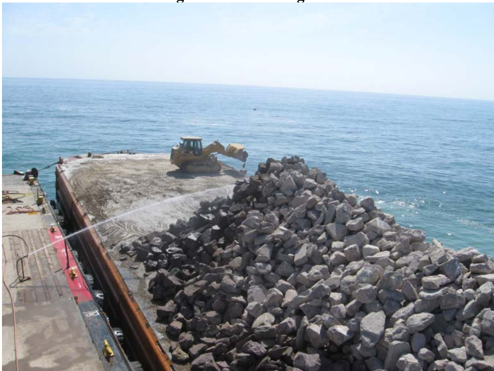
Photo G-18. Photograph taken on June 6, 2008, demonstrating how materials are placed and spread in the ocean.
