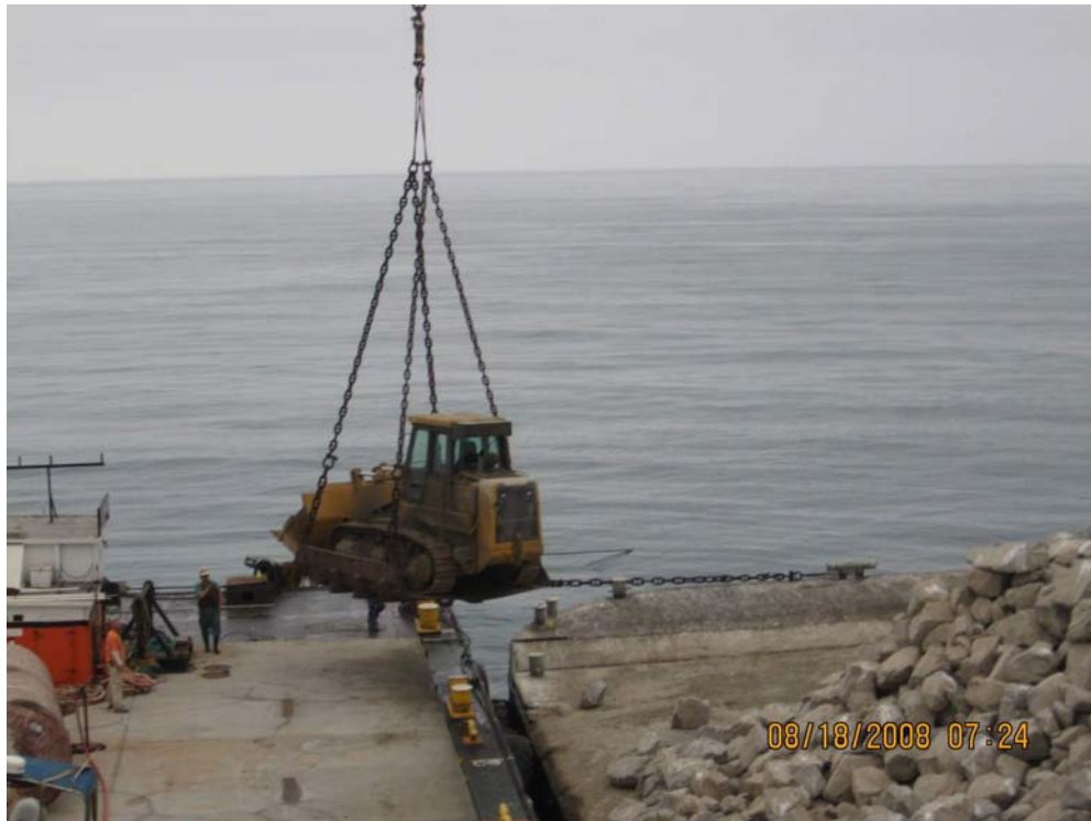
Photo G-17. Photograph taken on August 18, 2008, showing CP moving the truck loader from the derrick barge to the rock barge with a crane.
