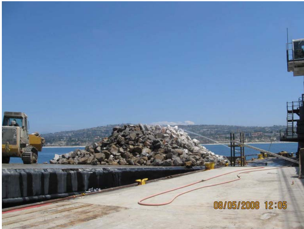
Photo G-19. Photograph taken on August 5, 2008, showing water being sprayed on the rock pile to reduce turbidity.
