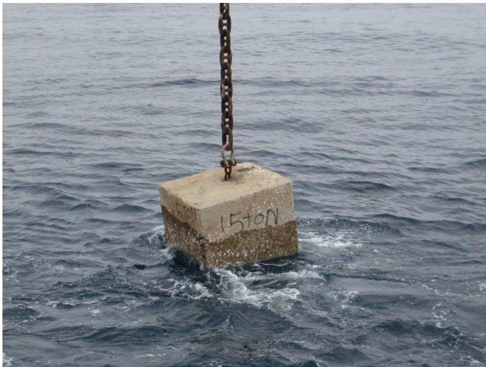
Photo G-12. Photograph taken on June 9, 2008, showing deployment of the 15-ton mooring block.
