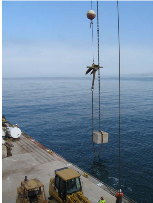
Photo G-11. Typical anchor system.
