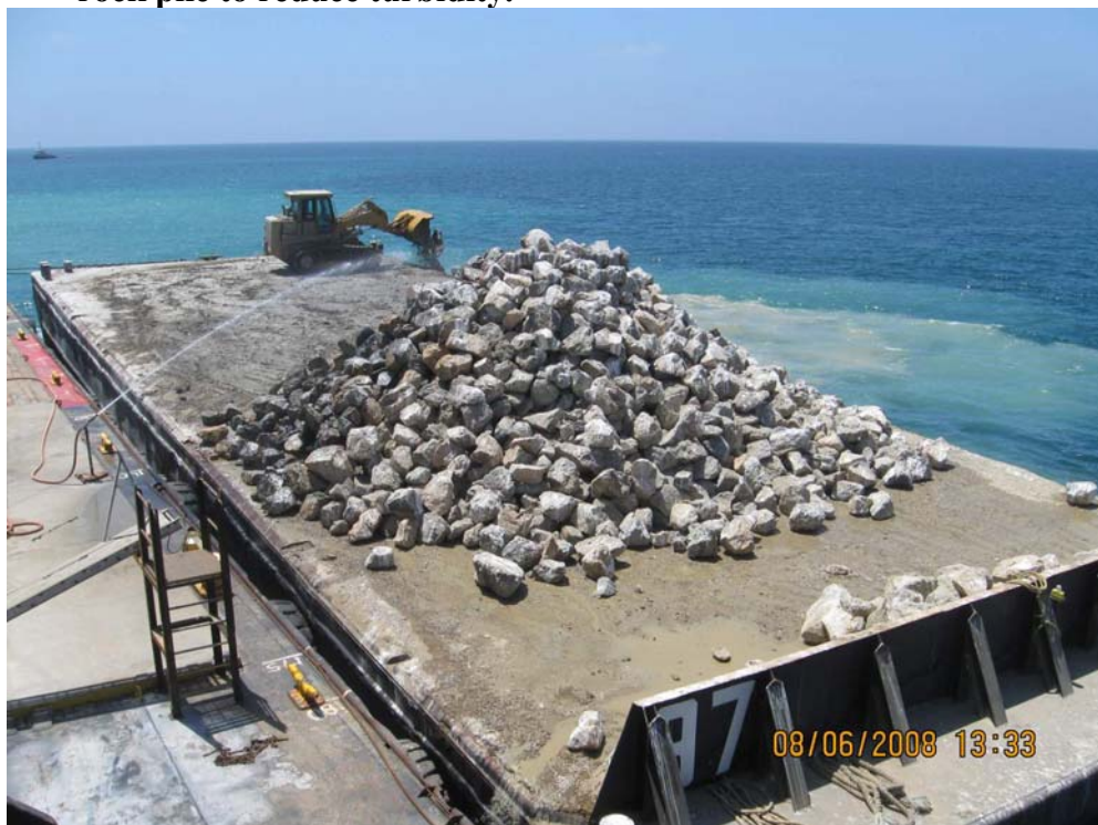
Photo G-20. Photograph taken on August 6, 2008, showing typical turbidity pattern caused by placing the rocks on the bottom of the ocean.
