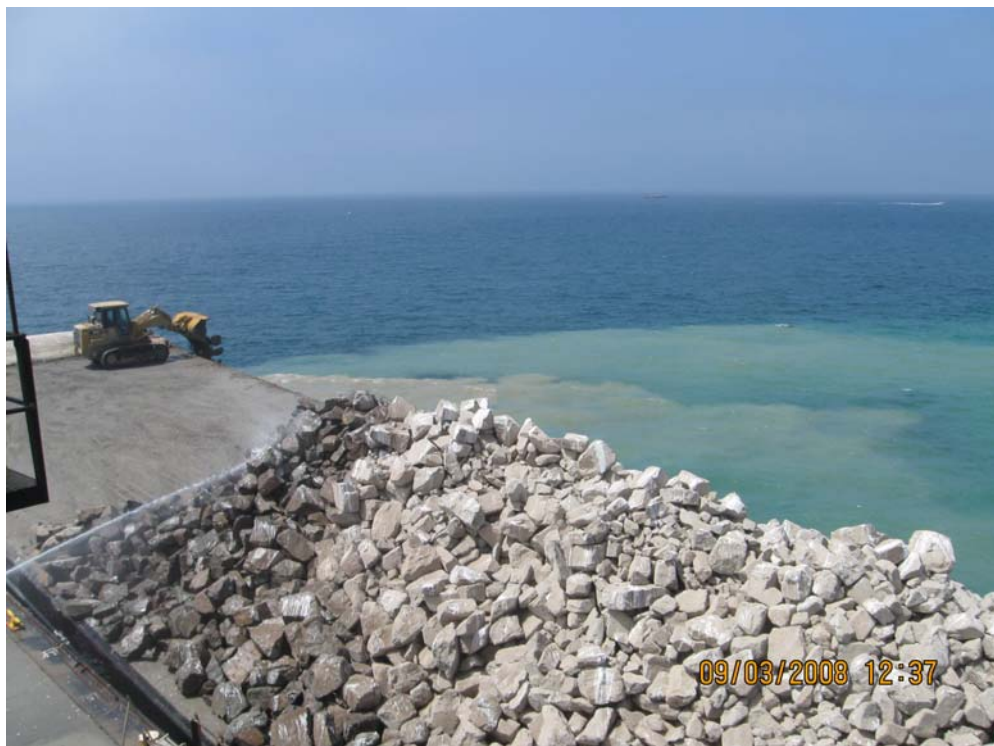
Photo C-14. Photograph showing average turbidity plume created during reef construction.
