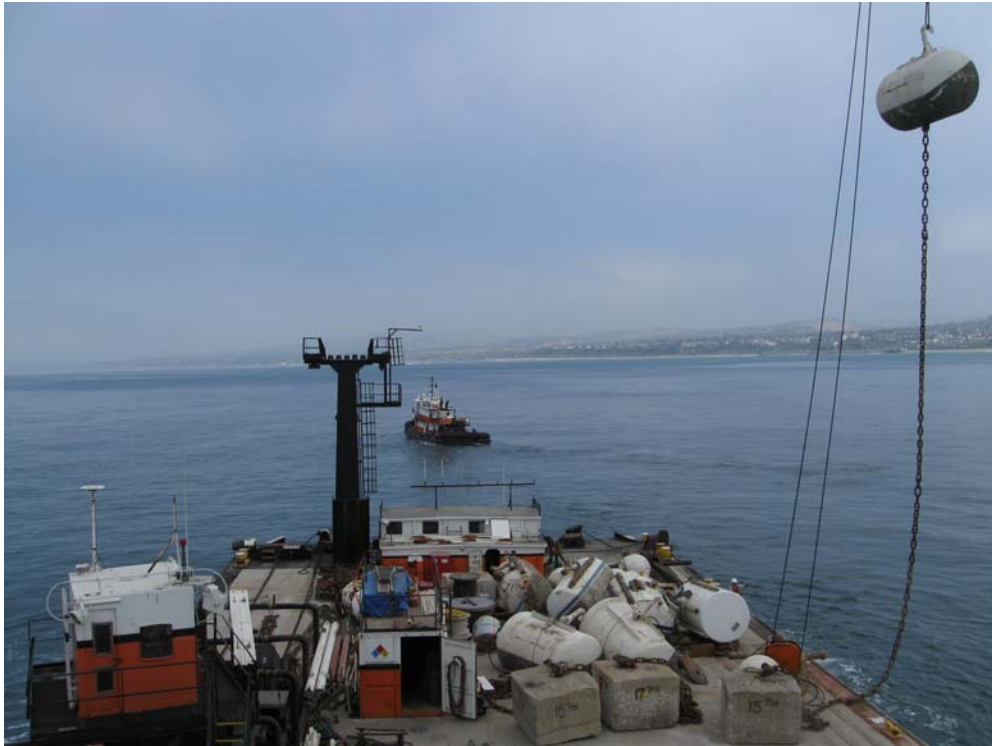
Photo C-5. Photograph showing anchor system consisting of surge cans connected to 15-ton concrete blocks and anchors. Anchors are beneath surge cans.
