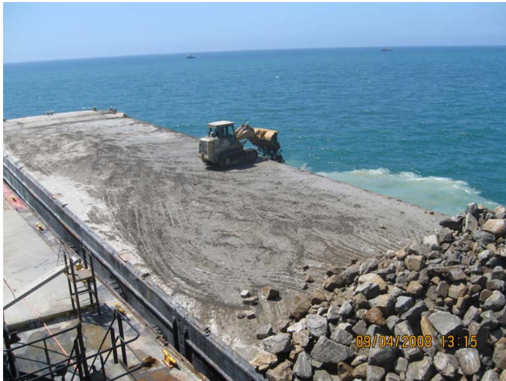
Photo C-11. Photograph showing rock placement by the front loader.
