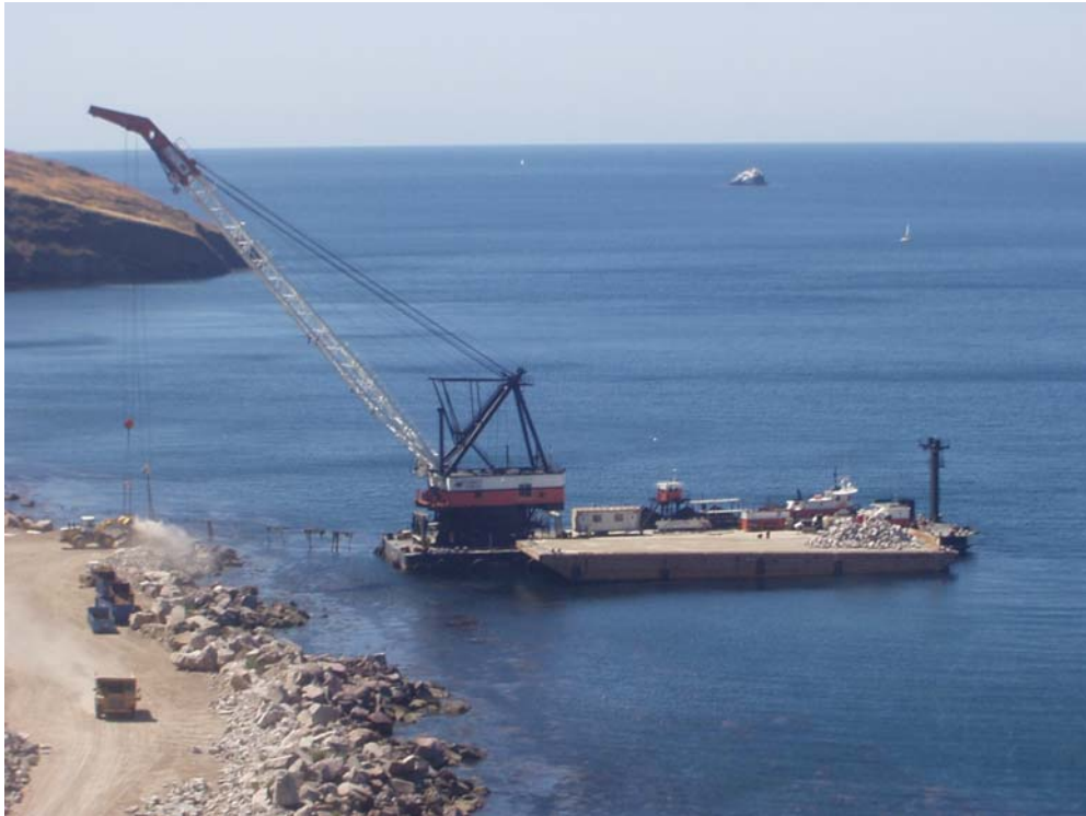
Photo C-3. Photograph showing derrick barge crane loading rocks from the Empire Quarry onto a rock barge.
