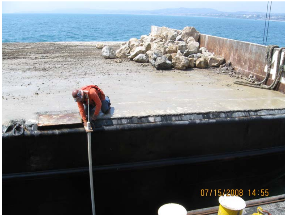
Photo C-13. Photograph showing construction worker measuring the height of the supply barge from the surface water at one of its four edges. Data is used to estimate the weight of the placed rock on the bottom of the ocean.
