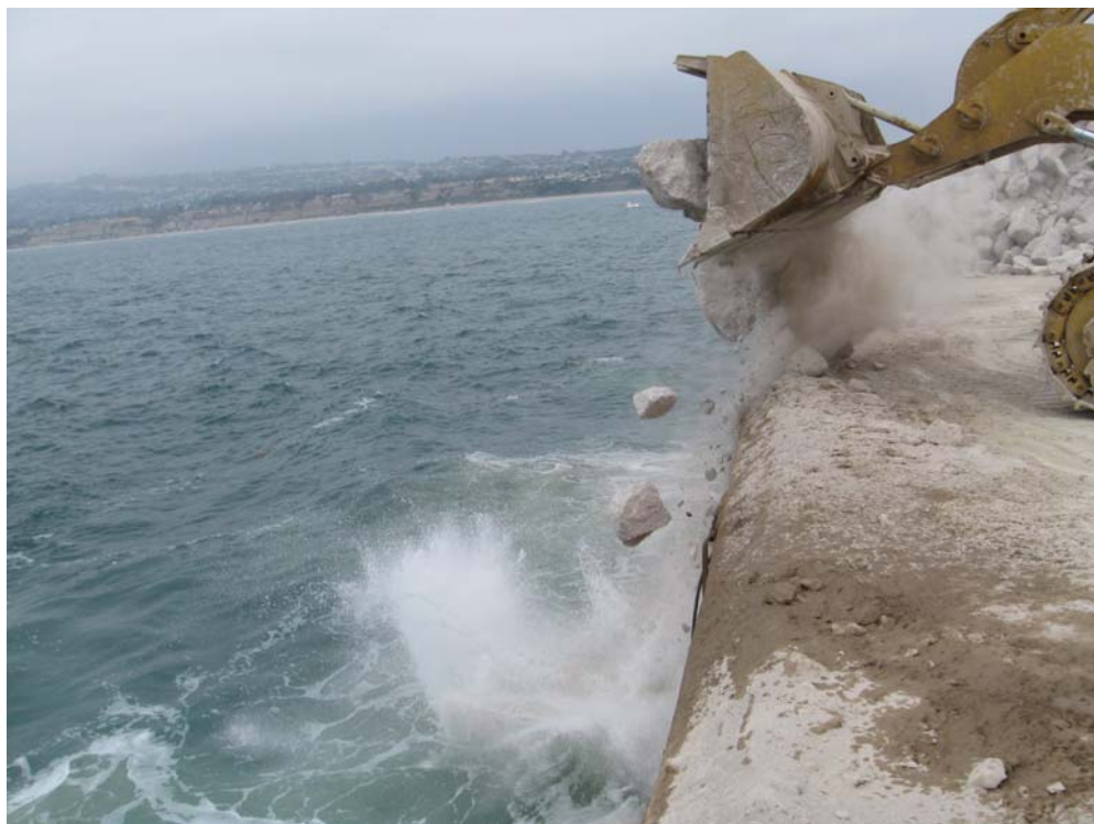
Photo C-12. Photograph showing a close-up view of rock placement.
