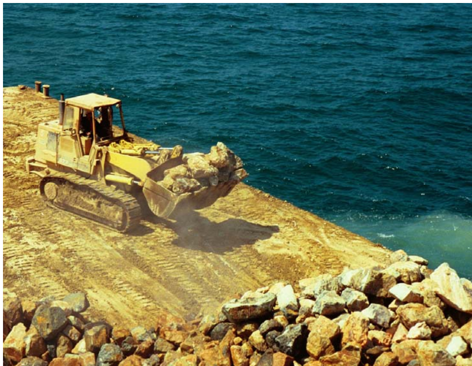
Figure 6-2. The Phase 2 Mitigation Reef rock placement method: The front-end-loader/flat-supply-barge “push off” method.
