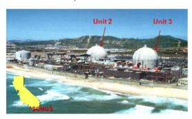
The nuclear reactors of SONGS units 2 and 3 were cooled by seawater that is taken in by large intake pipes and discharged back to the ocean via two diffuser lines
