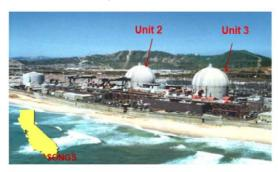
The nuclear reactors of SONGS units 2 and 3 were cooled by seawater that is taken in by large intake pipes and discharged back to the ocean via two diffuser lines
