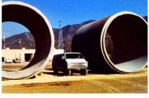
The nuclear reactors of SONGS units 2 and 3 were cooled by seawater that is taken in by large intake pipes and discharged back to the ocean via two diffuser lines
